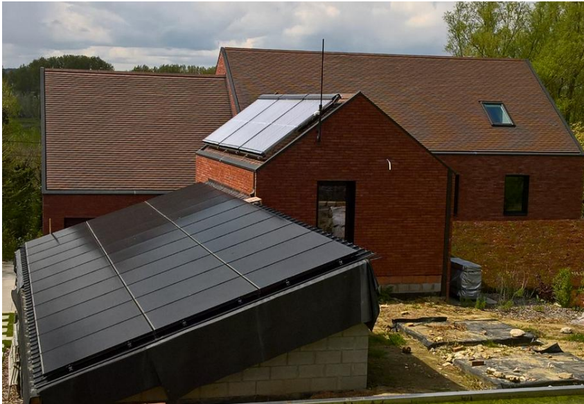
Figure 2 - A photo of the demonstration site: the residential building, large array of PV/T panels, three evacuated tube solar collectors and access to underground seasonal heat storages.
