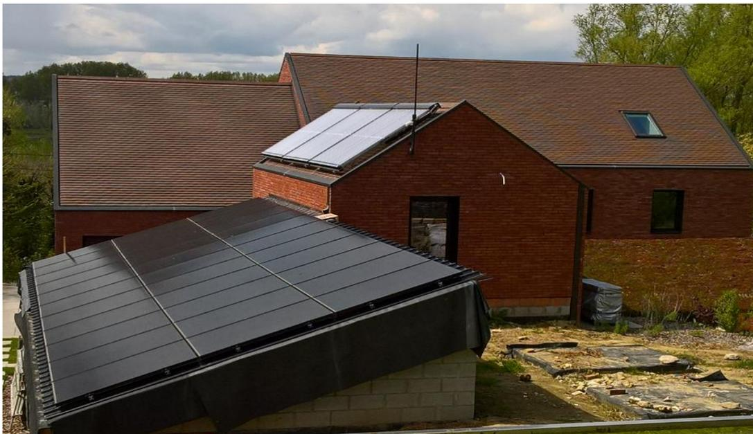
*Figure 1: A photo of the demonstration site: the residential building, large array of PV/T panels, three evacuated tube solar collectors and access to underground seasonal heat storages [1]*
