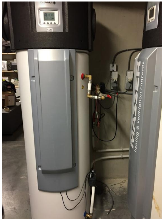
Figure 3. The 270-liter heat pump boiler controlled through LoRaWan.
