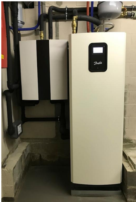
Figure 8. The Danfoss heat pump controlled through the ModBus- LoRaWan solution developed in the project.
