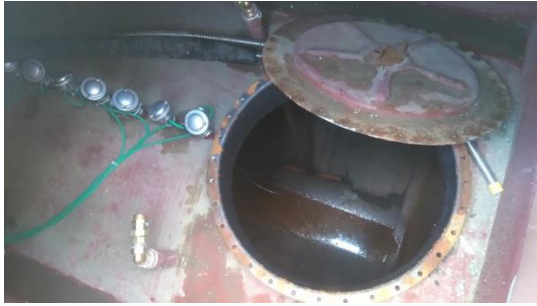
Figure 3: The picture shows the top of the tank, inside the small chamber before insulation is added. The stainless-steel heads with green wires connect the thermal sensors in the tank to a central management system. The tank is 2.5 m deep which equals the length at the top.
