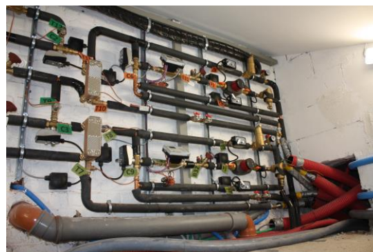
Figure 8: View on the 2 identical circuits connecting the heat exchangers with the vacuum boiler circuit with the two underground storage tanks. On the right is the exit to the underground tanks, on the left is the connection to the vacuum solar collector circuit.
