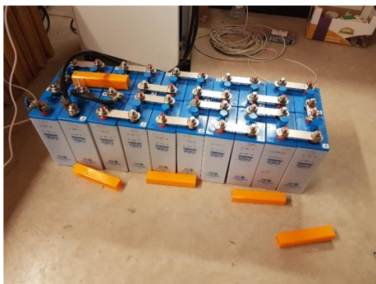
Figure 11: NiFe UPS system providing additional safety in case of a black out. Mainly relevant for preventing damage in very cold or relatively warm and/or sunny days. This battery system provides back-up power for pumps, valves and control in case the grid and the main battery system fail.
