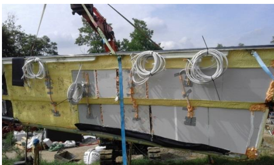
Figure 6: First cooling reservoir made of full epoxy vinyl ester resin with an armoured core of high performance fibres equipped with sensors before it is installed in the ground.
