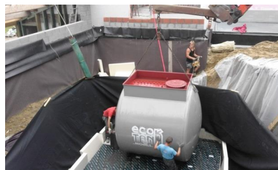
Figure 2: Putting the seasonal underground storage tanks in place. The tanks are installed in a large rubber bag filled with insulation. On the picture, the first tank is put in position.
