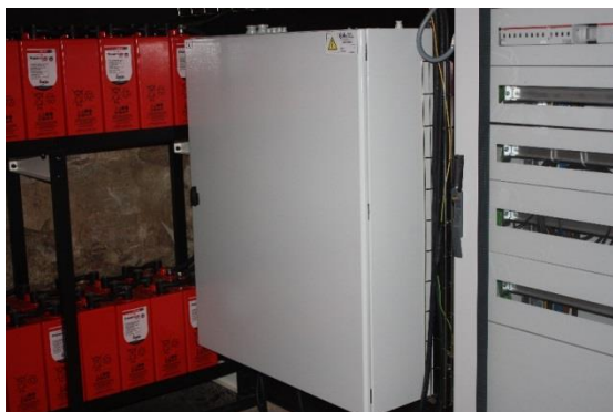
Figure 9: Lead-Acid batteries, 28 in total, providing 46.3 kWh full capacity, around 28 kWh of useful capacity. A large switchboard manages the smooth transition between off-grid and on-grid mode.
