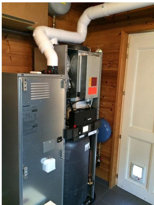
Figure 7: Inside of the device: left part is the fuel cell itself, right hand is the gas condensing boiler on the top and a thermal storage on the bottom.
