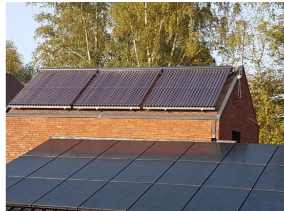
Figure 5: View on roof with vacuum solar thermal (upper roof) and PVT (lower roof) panels.
