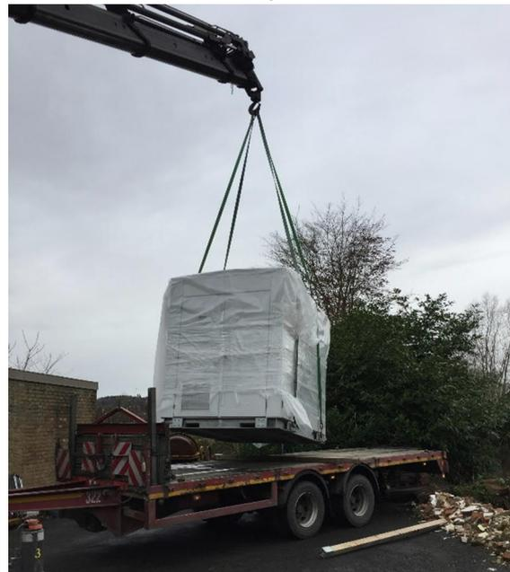
Figure 2 ABB Neighbourhood battery installation in Oud-Heverlee demonstration site
